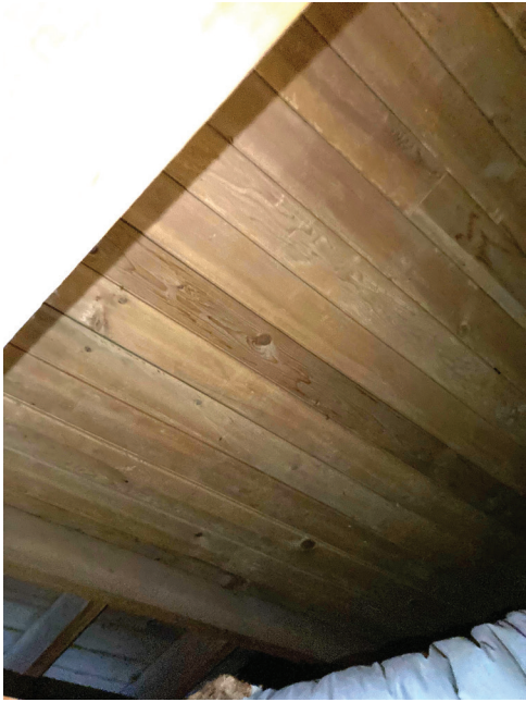
Current hidden ceiling under the drop tiles
