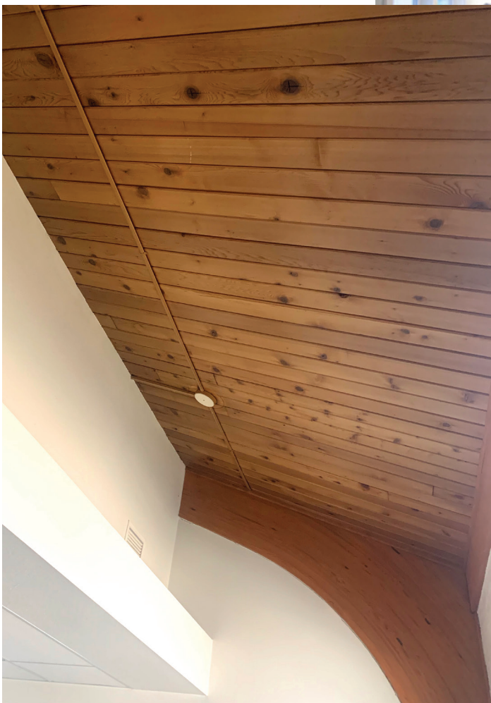
Current hidden ceiling under the drop tiles
